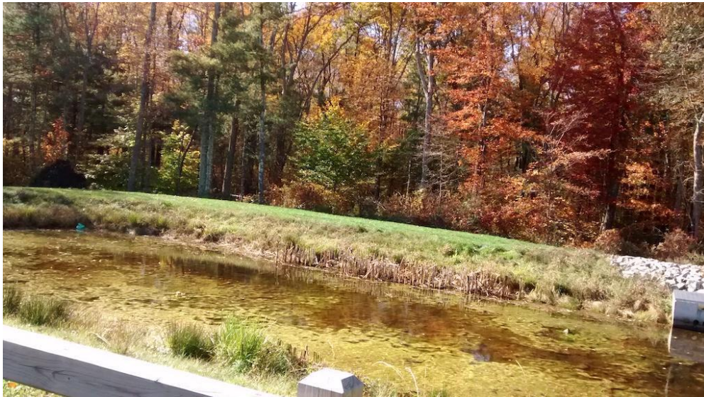
Figure 3b: Stormwater drainage on Lakeshore Center site with algae bloom (2023)
